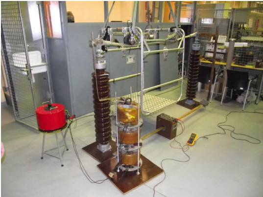
Figure 4. High current circuit in the High Voltage Laboratory of BUTE.
